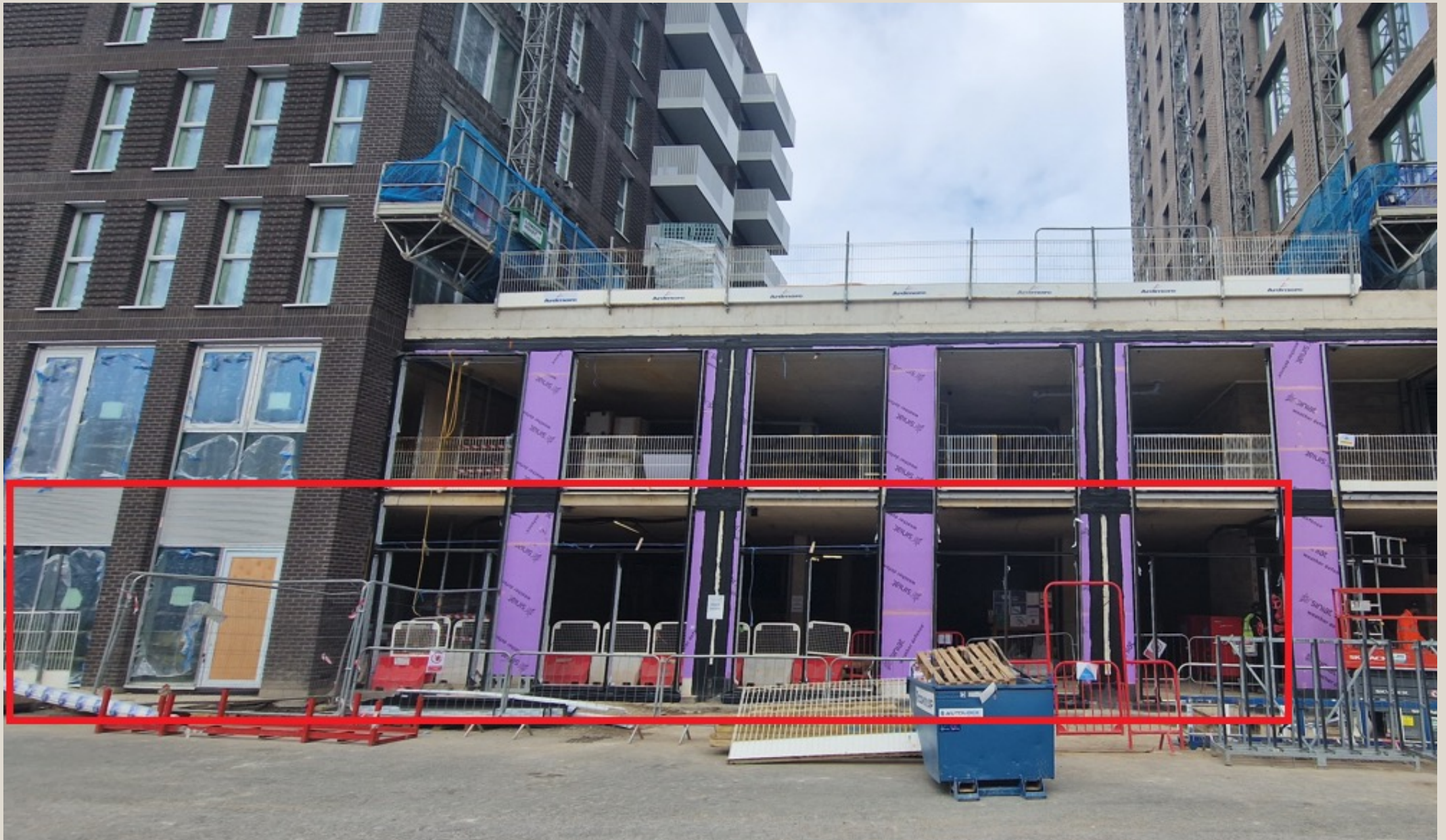
Image showing the unit under construction. Taken April 2023.
